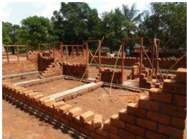
A new house going up
