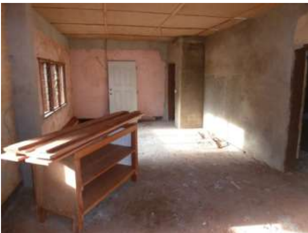
Living room of a house during renovation
